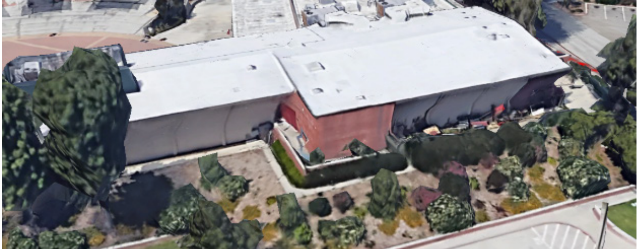
Figure 25: Example of oblique images showing sides of buildings, where CTs can sometimes be located.
