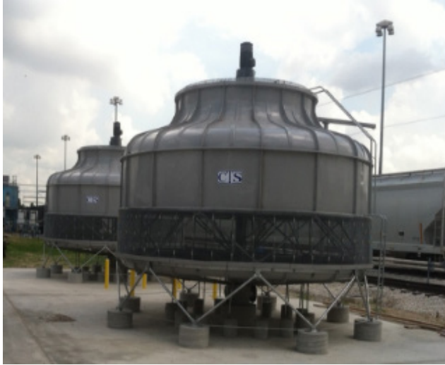
Figure 6: Round designs of open CTs, often substantially smaller than other CTs and more commonly on the ground. (Images of branded CTs courtesy of Delta Cooling Towers and Cooling Tower Systems .)
