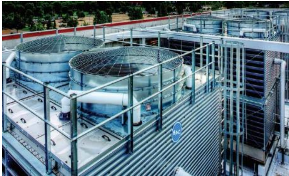
Figure 5: Rectangular and square CTs, the most common types of CT. (Images of branded CTs courtesy of Delta Cooling Towers and SPX Cooling Technologies .)
