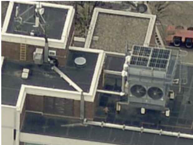
Figure 8: CTs with side fans or other less common fan configurations.
