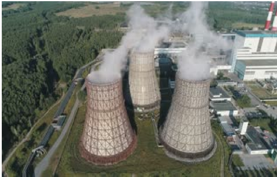
Figure 7: Large hyperboloid shaped CTs are typically easy to find on a satellite images but are much less common; these models are used for very large industrial plants.
