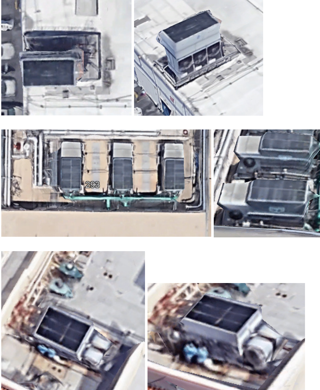
Figure 13: Oblique images reveal side fans. CTs with side fans are easy to miss but generally have characteristic dark grated tops and otherwise retain the same characteristics as other CTs (building types, pipes, logos), though fan diameters tend to be smaller than other CTs (less than 2m). High index of suspicion is needed to identify these.
