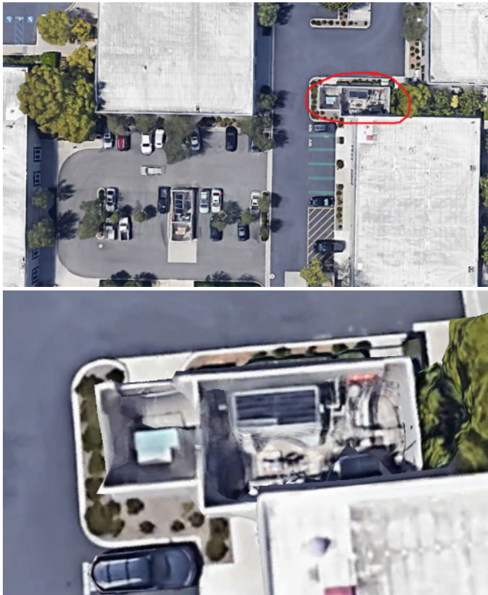
Figure 5: A lack of A/C for warehouse area buildings is suspicious (exceptions of course depending on what is being stored there). On closer inspection, the CT is found (Top, red circle) with zoom of area (bottom).
