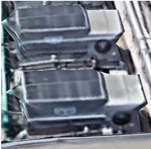
Figure 15: CTs are often branded with the company logo, which can be helpful for identification. Two distinctive, popular brands are BAC (top) and evapco (bottom).
