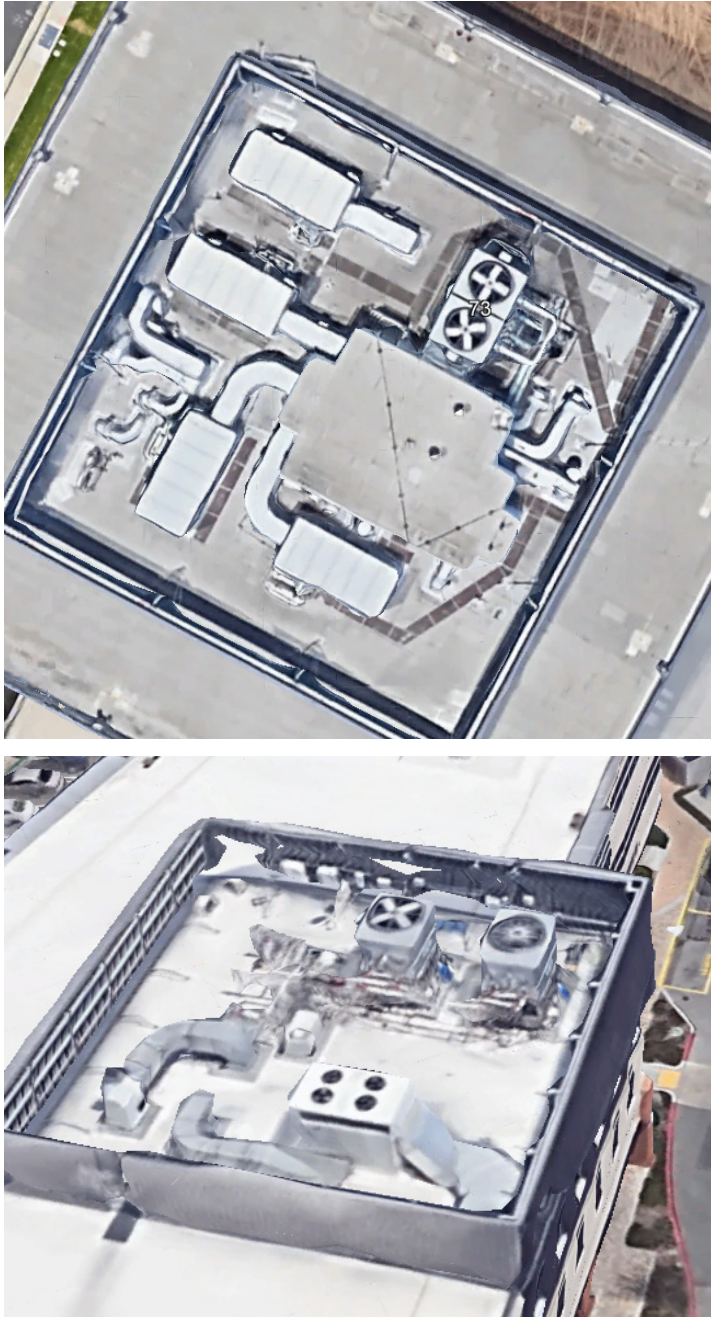
Figure 6: Two CTs (labeled 73) with multiple water white water pipes versus four non-CTs with large air ducts (CTs circulate water to and from the building, not air; top image). Two CTs (top of picture) with multiple small pipes and non-CT with small fans and a large air duct running to it (bottom image).
