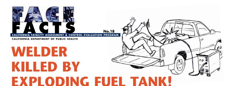
In a recent incident, a twenty-five-year-old welder, Carlos S.\*, died while repairing a fuel tank. The tank was attached to the bed of a pick-up truck. There was still some flammable liquid or vapor left in the tank when Carlos started welding. Carlos had never had classes or other formal training in welding safety.
