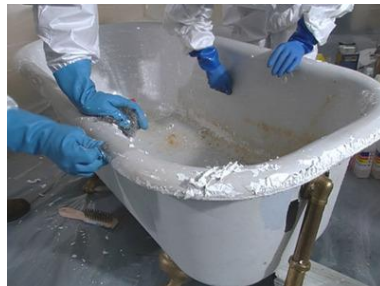
Workers using a MeCl-based stripper to remove paint from a bathtub prior to refinishing.
