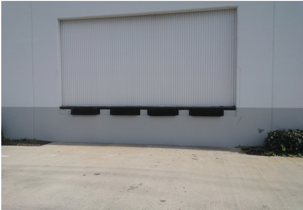
Exhibit 1. A truck loading dock identical to the one involved in the incident. Trucks back up to the dock in order to load and unload product.
