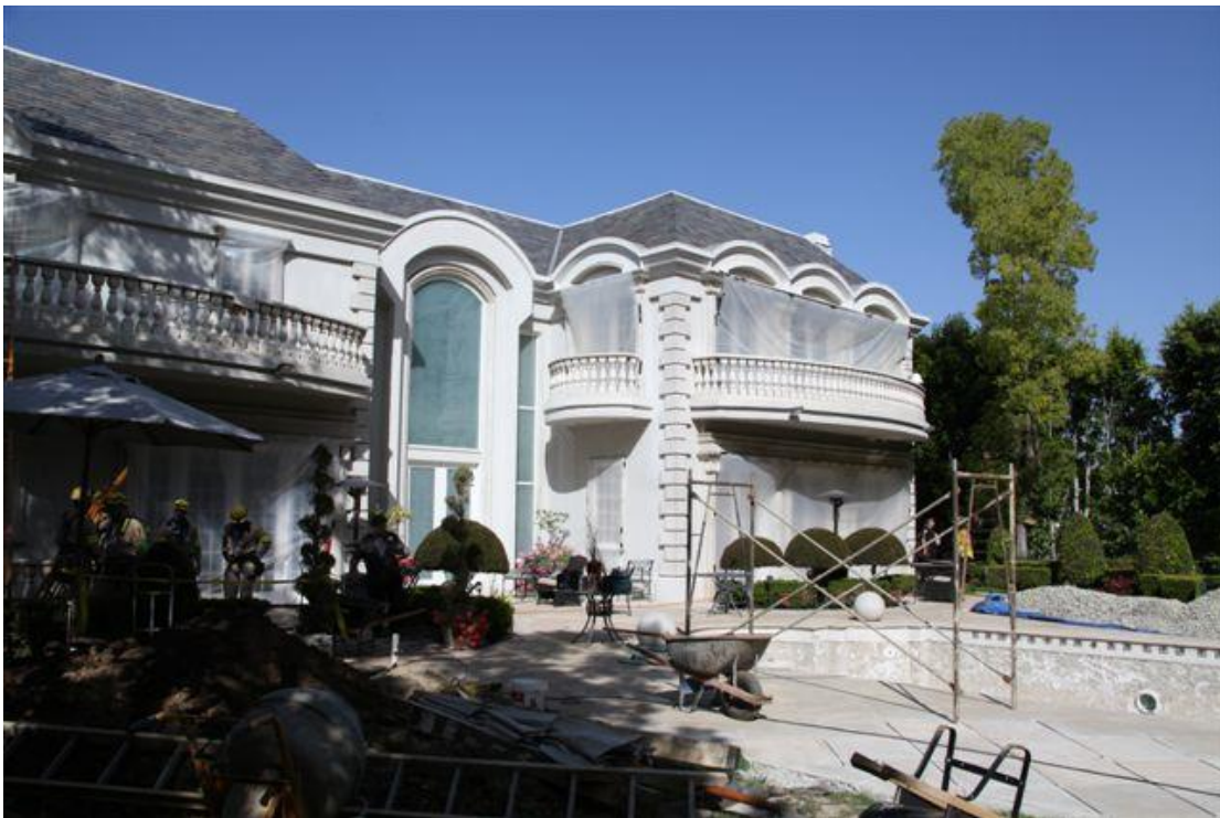
Exhibit 1. The back yard and rear of house where the incident occurred.
