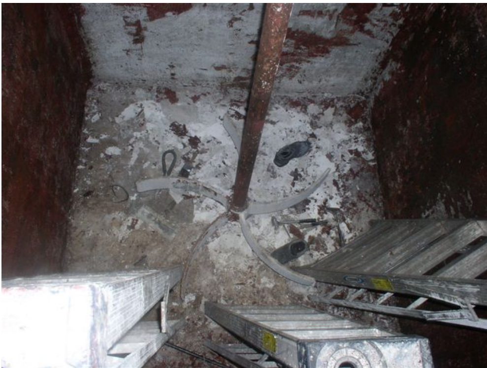
Exhibit 5 – The ladders used to enter the tank.
