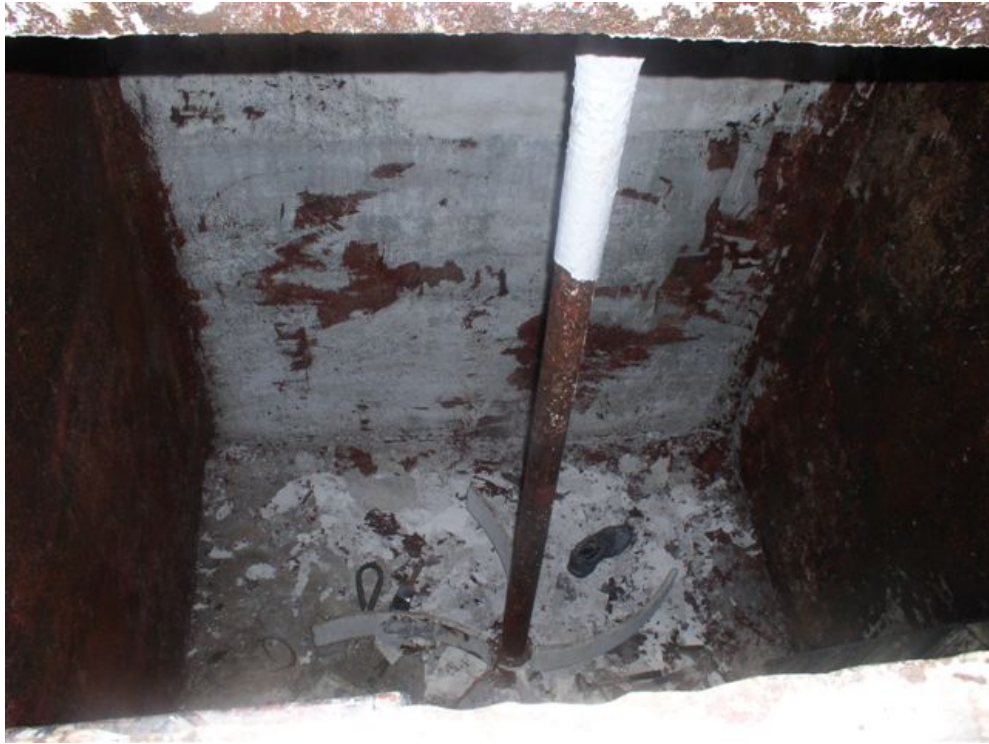
Exhibit 4 - The interior of the paint tank.
