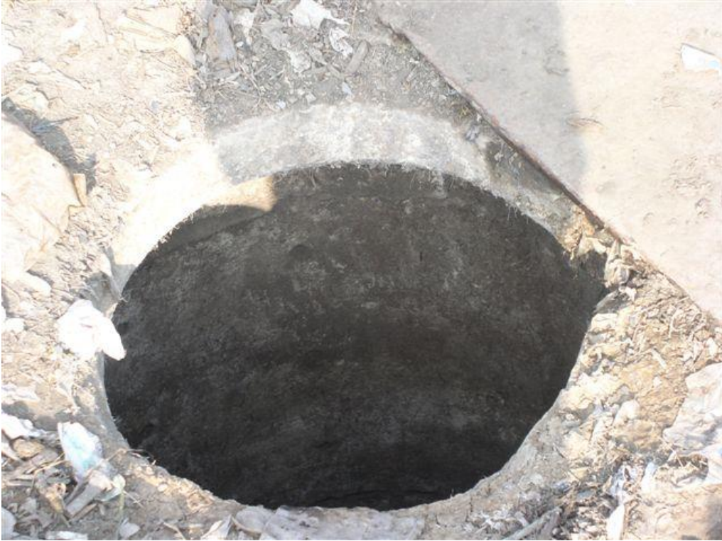
Exhibit 4. A close-up of the shaft opening.
