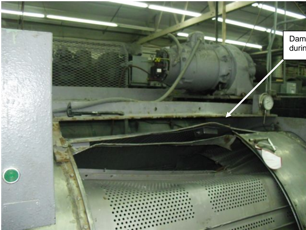
Exhibit 4. The industrial washing machine opening.
