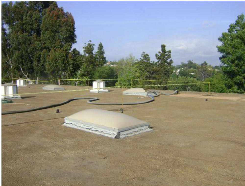
Exhibit 2. The work area on the roof.
