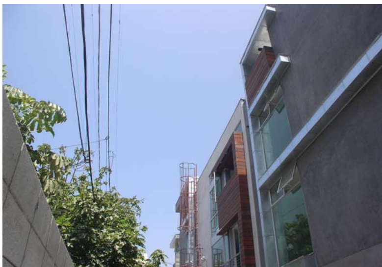
Exhibit 2. The top of the building under construction where the victim was working.
