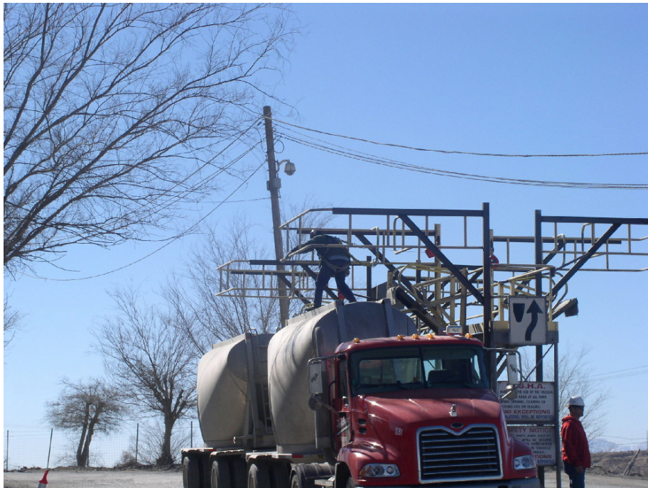
Exhibit 4. An employee using the catwalk and gangway to gain access to the top of a tanker trailer to close the lid.
