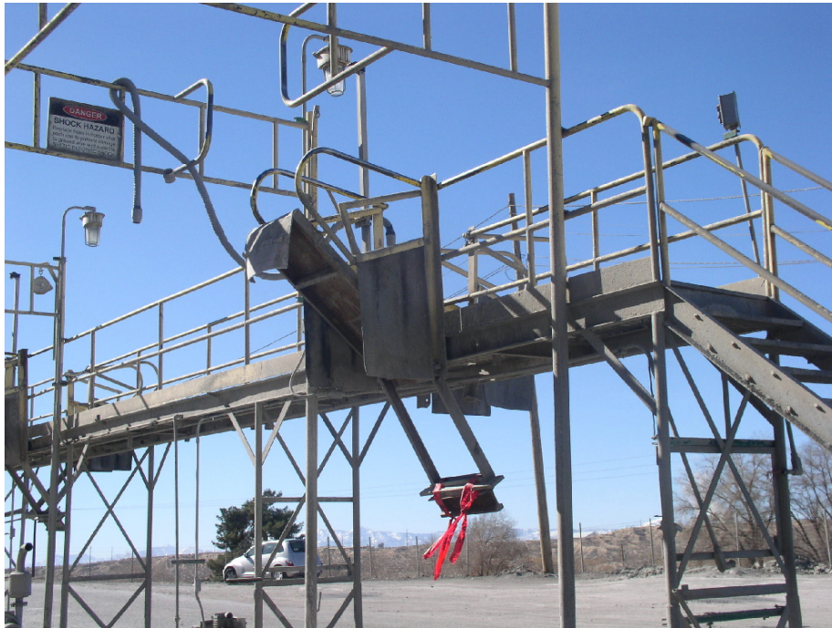
Exhibit 3. The weighted gangway and safety guardrail that extends over the top of tank trailers parked below.
