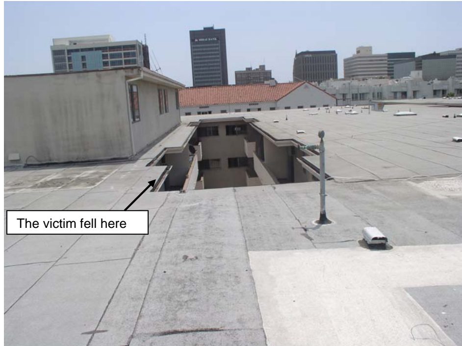
Exhibit 3. The roof opening where the victim fell.
