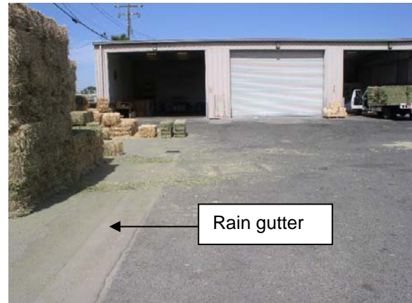
Exhibit 4. The rain gutter built into the asphalt yard.
