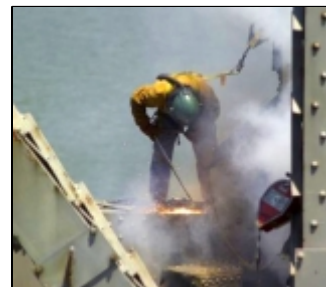
Photo: Demolition worker disturbing old lead paint
