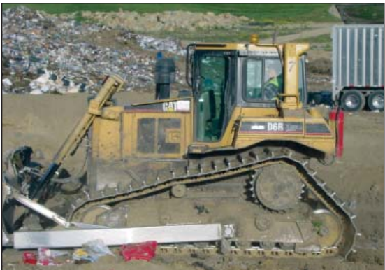
Figure 28. Bulldozing treated medical waste at landfill
