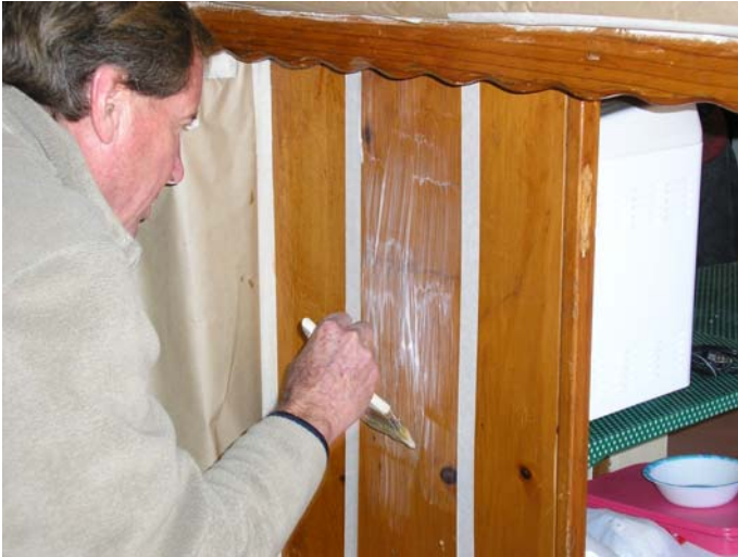
Figure 6-2. Brushing Stripper on Panel
